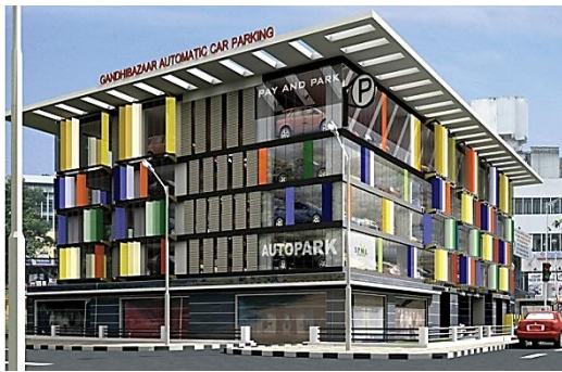
Fig 15 the entire automated parking unit.
